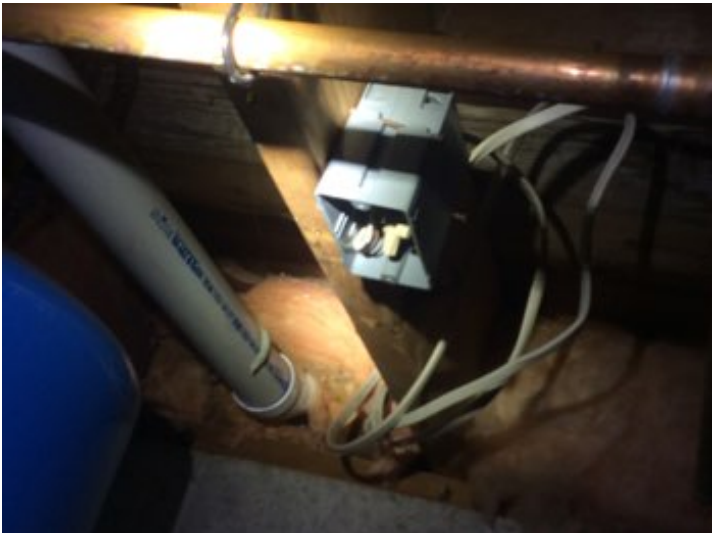
Missing electrical junction box cover should be installed
