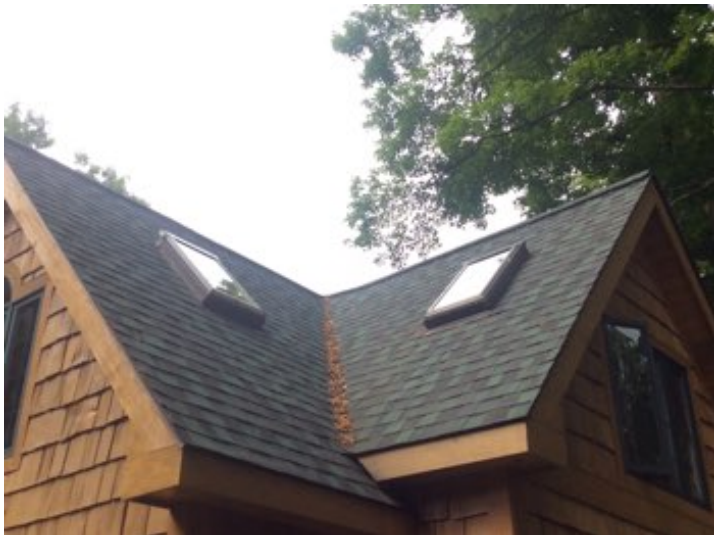
NE side of the outbuilding. We recommend cleaning off tree debris as it can hold moisture to shingles causing premature decay and a shortened shingle service life.
