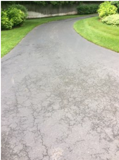
Asphalt driveway-We recommend sealing any small cracks in drive to prevent further expansion.
