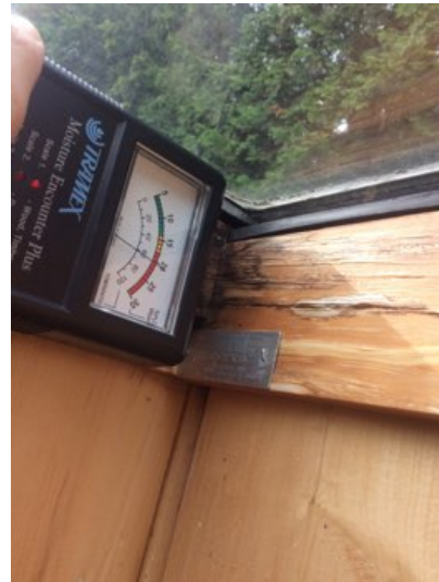
Staining at the gym skylight window tested slightly damp at time of inspection with moisture meter. We recommend a qualified contractor evaluate and repair as needed.
