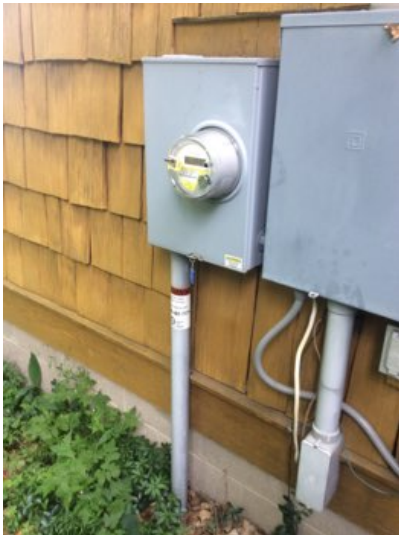
Lateral electrical service appears secure
