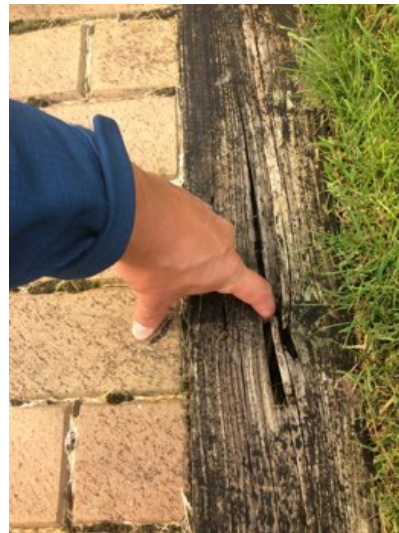
N brick water walkway-multiple landscaping timbers observed to have decayed areas, we recommend replacing to prevent bricks from settling/shifting.
