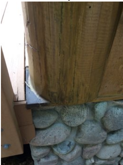
Decayed corner beam observed at NW corner of home.
