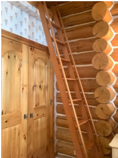
N bedroom: we recommend properly securing loft ladder to improve safety
