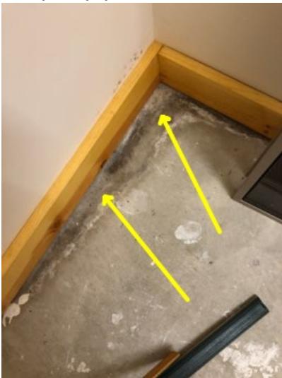
North east storage room near crock: concrete floor has water staining with hard water deposits. Although the area was dry during inspection this is an indication of repeated wetting. We recommend consulting with seller for history of water intrusion
