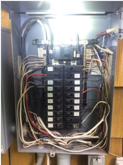
100 amp service, copper main conductors. Breakers and wiring appear secure. Panel appears to be properly grounded.
