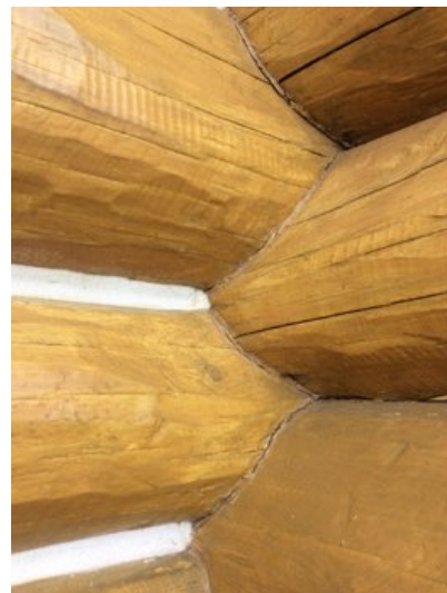
We recommend sealing any cracks in or around logs to prevent water damage and further expansion.
