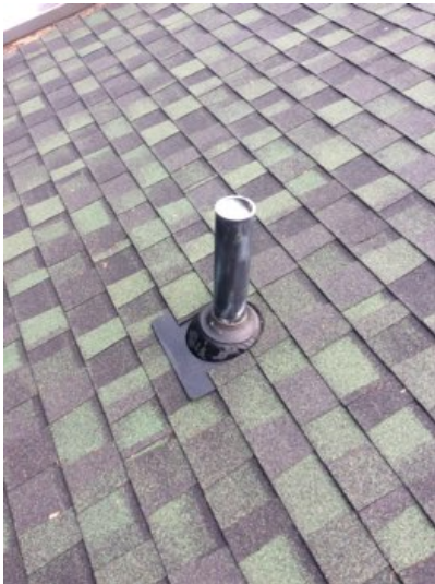
Lower SW waste vent appears secure
