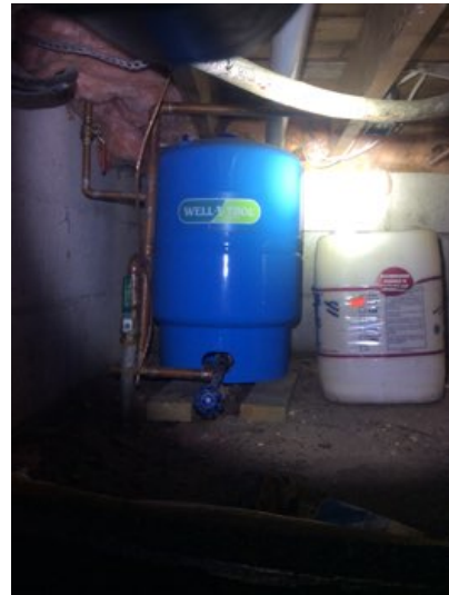
Pressure tank and water shut-off appear secure, located in the NE corner of the crawlspace
