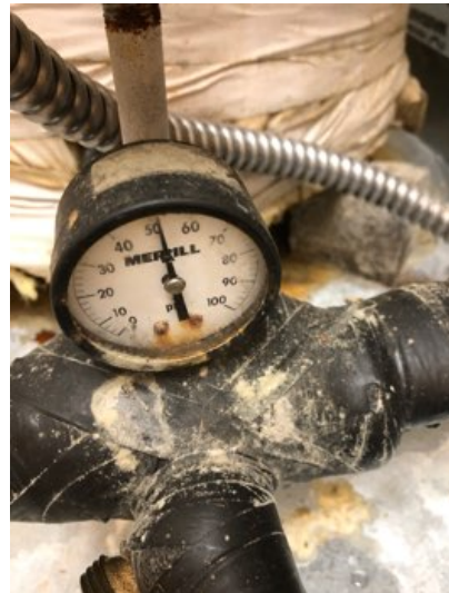
Although the well appeared to cycle properly and good water pressure was observed throughout the home, pressure gauge did not function. We do recommend replacing the pressure gauge to get an accurate pressure reading.
