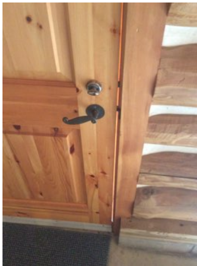
Weather stripping at service door should be improved
