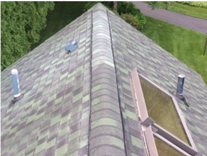
Upper SE waste vents appear secure. We recommend resealing face nails in flashing to prevent water intrusion.
