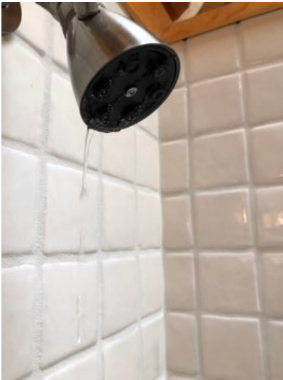
Showerhead drips, may need a new diverter valve in faucet
