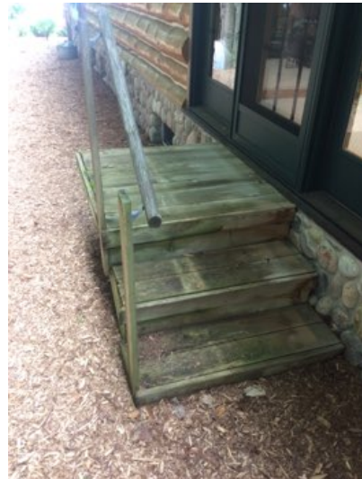
W side entry deck-deck boards/trim starting to decay and hand rail loose and should be replaced.
