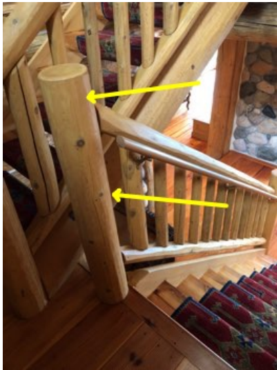
West lower railing is slightly loose and should be secured
