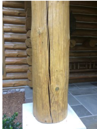
We recommend sealing any cracks in logs to prevent water damage and further expansion.
