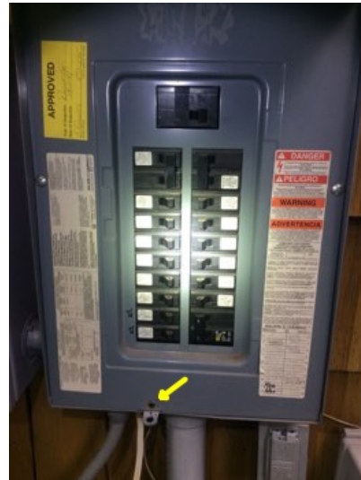
Outbuilding service panel ledger appears to be complete. Missing panel cover screw should be installed.
