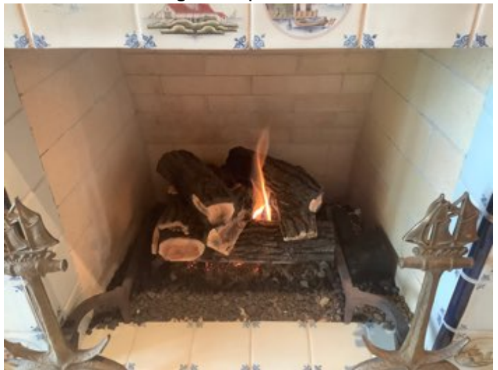
W living area: gas burning fireplace tested and functioned properly. We recommend installing some sort of door or cover for fireplace.
