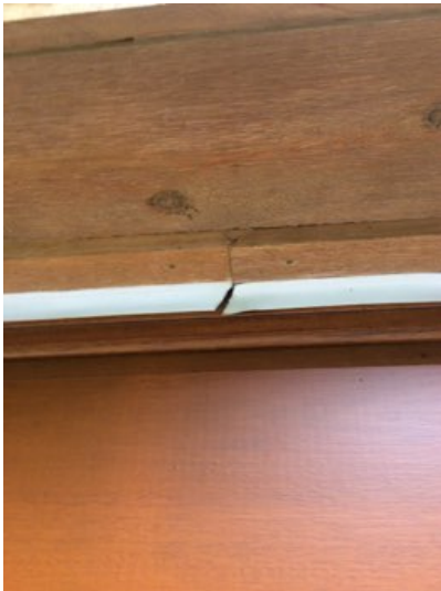
Seam in garage door weather stripping should be sealed to prevent water intrusion.
