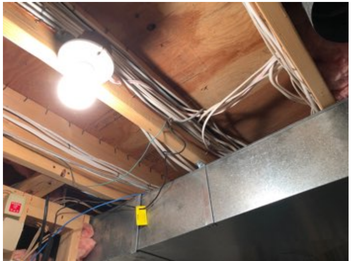
2 x 10 floor joist construction on 16 inch centers
