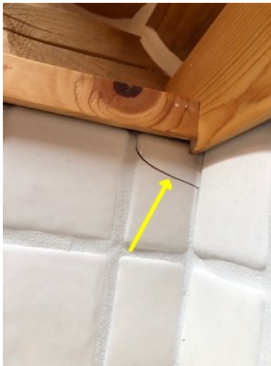
Cracked tile in tub/shower upper corner
