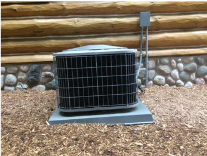
Carrier A/C condenser with electrical shutoff present
