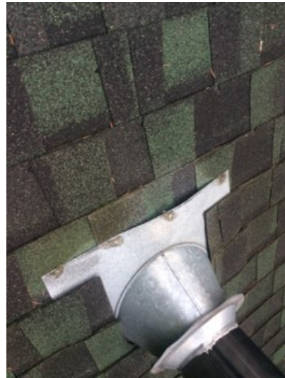
Lifted flashing of the lower NE vent stack should be secured to prevent water intrusion
