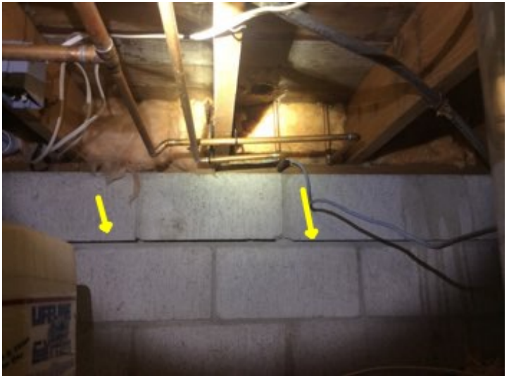
Cracking and slight gap in tuck pointing at the NE corner of the crawlspace. We recommend a qualified contractor evaluate and seal gap for further monitoring.
