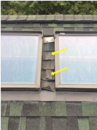
Decayed shingles between the upper SE skylights should be replaced
