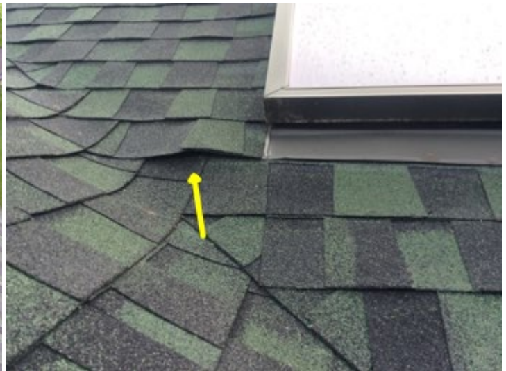
Lifted shingle/flashing at the upper SE skylight should be secured to prevent water intrusion and wind damage
