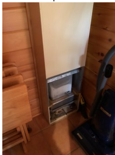
Gas wall heater, unit responded to thermostat, located on kitchen wall
