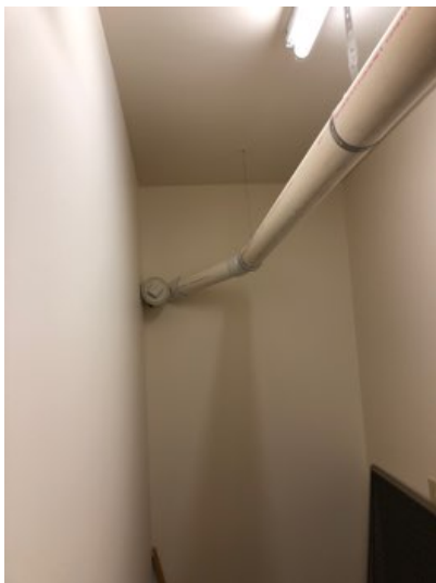
Visible waste line is adequately supported
