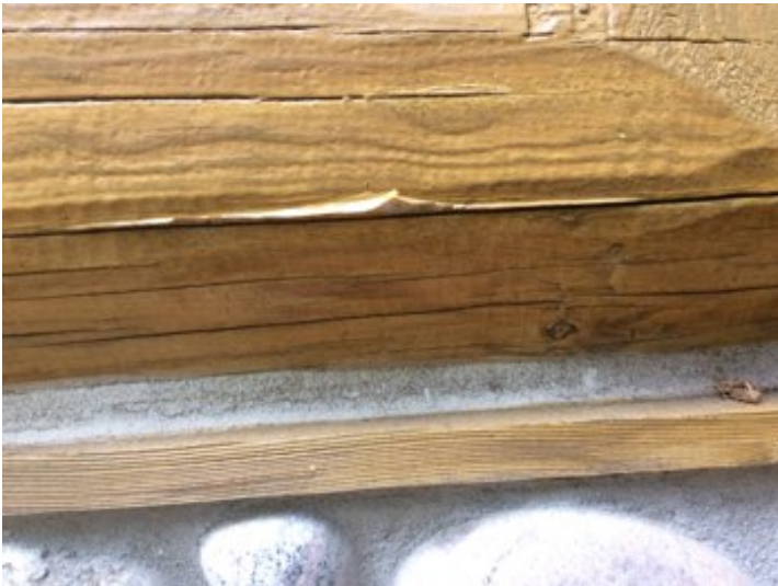
Chipping sealant observed at lower SE corner. We recommend scraping and resealing these areas to prevent water damage.
