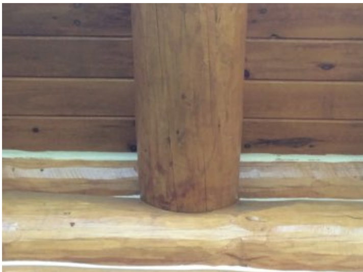
Cracked chinking observed above NW living room windows should be resealed to prevent water intrusion.
