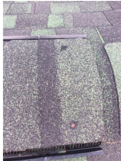
We recommend resealing face nailing at the end of ridge run shingles to prevent water intrusion.
