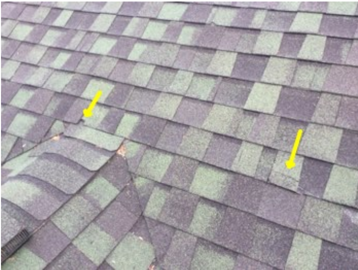
Ripped shingles near the upper S side ridge should be replaced to prevent water intrusion
