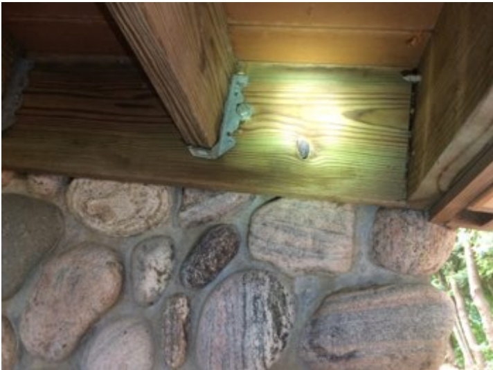
NW Deck 2x8 construction on 16" centers with 6x6 supports. Ledger board is bolted and not flashed. We recommend properly flashing the ledger board for improved deck safety.
