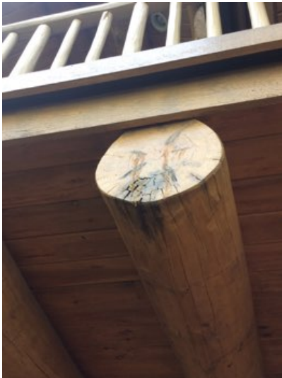
Decayed log tail observed on underside of upper NW deck.
