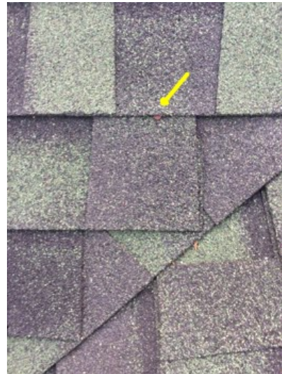
Exposed nail in the W valley of the upper NE dormer should be sealed to prevent water intrusion
