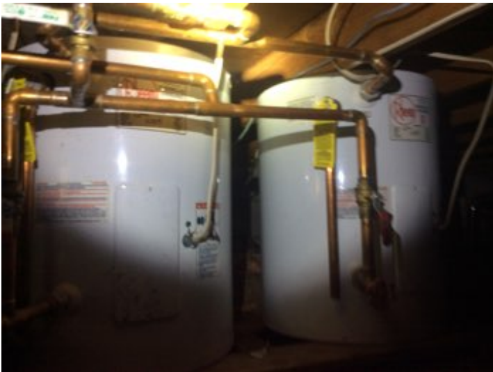
2-Rheem 19.9 gallon electric water heaters. Units responded to hot water testing. Average service life of a hot water heater is 5-15 years.
