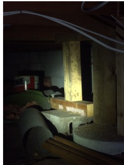
Improperly set block support should be adjusted. We recommend a qualified contractor evaluate and repair as needed to improve support.
