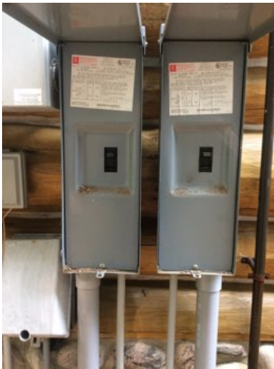
Dual exterior 200 amp service mains
