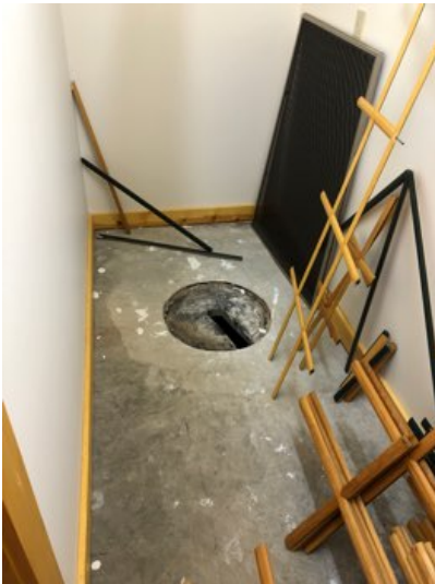
North east storage room: a crock has been installed, no pump present, inside crock is dry
