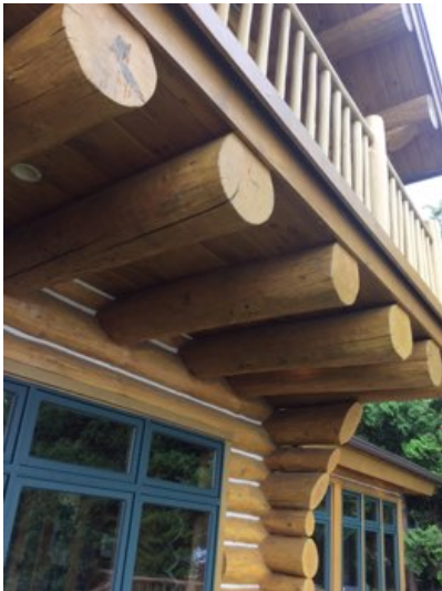
Upper NW deck-Log cantilevered construction appears secure.
