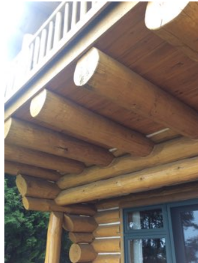
Upper NE deck-Log cantilevered construction appears secure.
