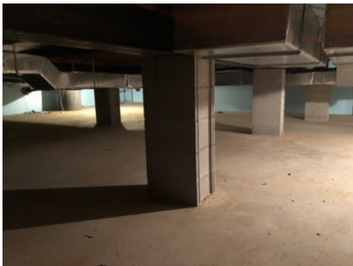
Crawl Southview: Concrete block column supports are secure floor joists are supported with steel I-beams. Exterior walls are insulated with 1 inch foam board
