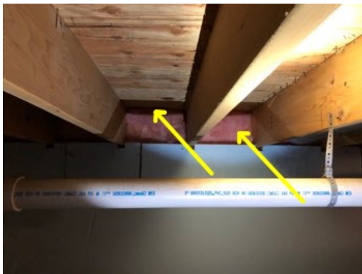
Crawl space: visible rim joists are insulated
