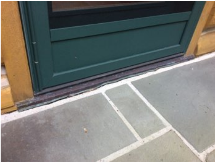
We recommend sealing the crack at the base of S side entry door to prevent water intrusion.
