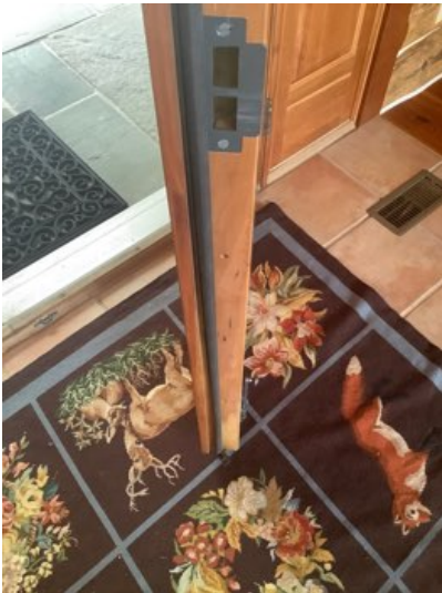
Front entryway: we recommend securing weatherstripping on right door and sealing grout cracks at door threshold.
