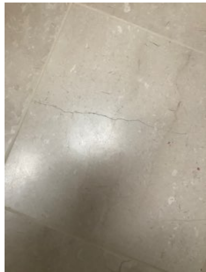
Crack observed in tile
