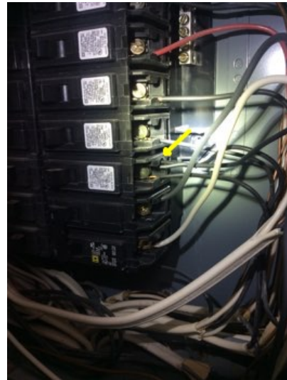
Outbuilding service panel: Double tapped breaker(s) inside panel box (more than one electrical conductor attached). This is not standard practice, and may cause overheating or even an electrical fire. Recommend evaluation by an electrician. Double tapping and lugging can create hot spots on breakers and neutral bars because they are not tightened to the correct torque--especially if two different size conductors are used. Because the hot [black] and neutral [white] wires are both current carrying conductors, the chance is then greater for potential hot spots. If the double tap or lug becomes loose, it begins to arc. As it arcs it builds up carbon. Carbon is then resistance and with more carbon buildup the more difficult it is for the conductor to make contact, thus increasing the current. The end result can be the breaker tripping because of the loose connection [current exceeding the rating of the breaker], or signs of overheating such as discolored wires, melted wires, etc, or even fire.
