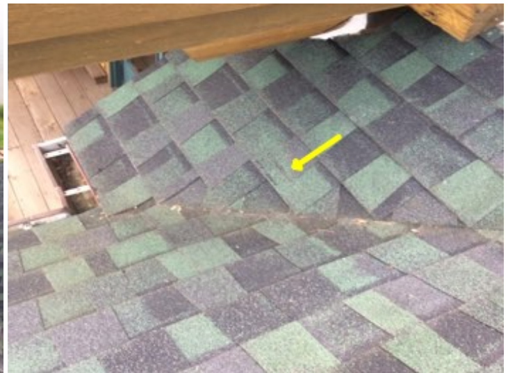
Ripped shingle at the bottom of the E valley of the upper N side should be replaced
