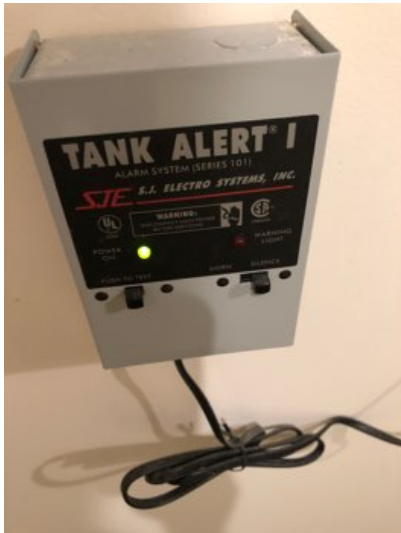
Septic tank alert sounded when tested
