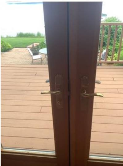
E living area: left and right N exterior doors don't latch properly, but do lock. We recommend adjusting.
